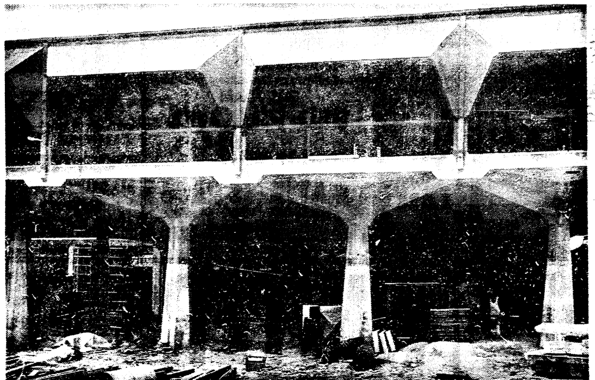
POURED-IN-PLACE CONCRETE posts were topped with concrete prongs to support the second floor of the new Pioneer Broadcasting Co. building at 1501 SW Jefferson St., designed by Fred Bassetti & Associates, Seattle. The
