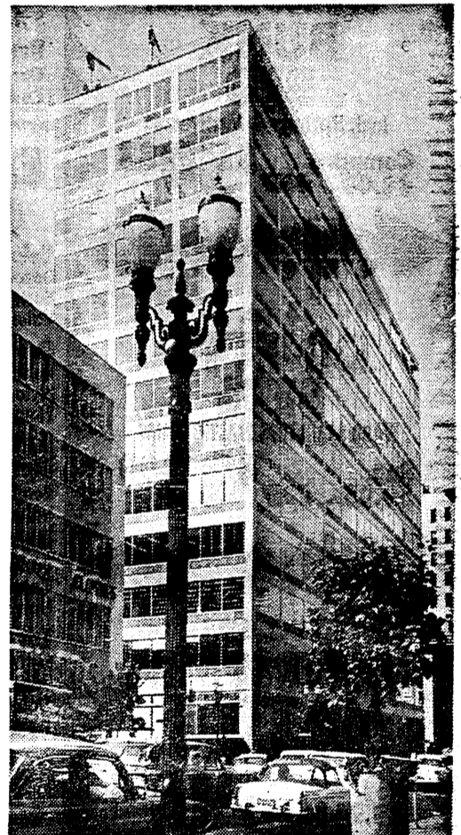
ONE OF THE NATION'S first glass-walled office buildings was Equitable Savings & Loan Association, 421 SW 6th Ave., designed by Pietro Belluschi and constructed after World War II. The tower served as a model for smooth-surfaced buildings and helped to establish an international trend. Architects now seek more decoration and variety of materials.
