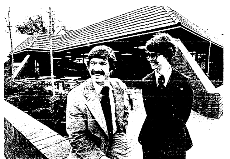
DOWNTOWN DRESS — Strict standards of design for the Portland core area resulted in a more elaborate and costlier building for a new downtown Burger King fast food restaurant. Franchiser Joseph Angel stands in front of the structure with his manager, Nancy Franklin.
